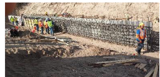
Border wall under construction
