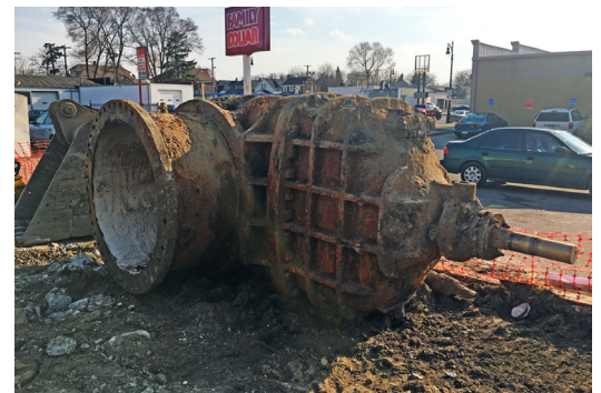
Broken (Frozen) Valve After Removal.
