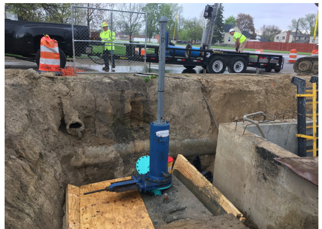
LGC Crew removing concrete encasement from the 24" pipe to install the line stop. Location is Marquette & Inkster, Detroit.
