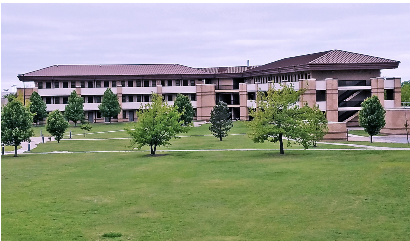
One of 3 Airmen's Dormitories at McConnell Air Force Base - Wichita, KS.
