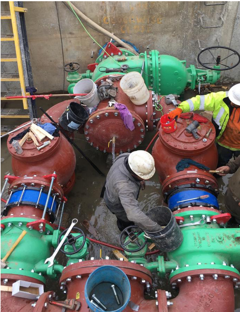
Pressure regulating valve vault improvements. Marquette & Inkster in Garden City, MI. Two 16" PRO'S and piping connected through 24" pipe to 30" and 54" water transmission main. This PRV vault controls the pressure from higher zone to intermediate pressure zone.
