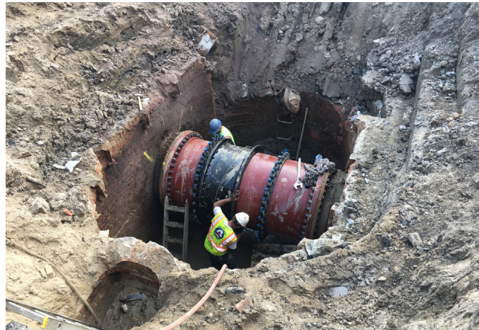
LGC Crew installing 48" piping after removing broken frozen valve.
