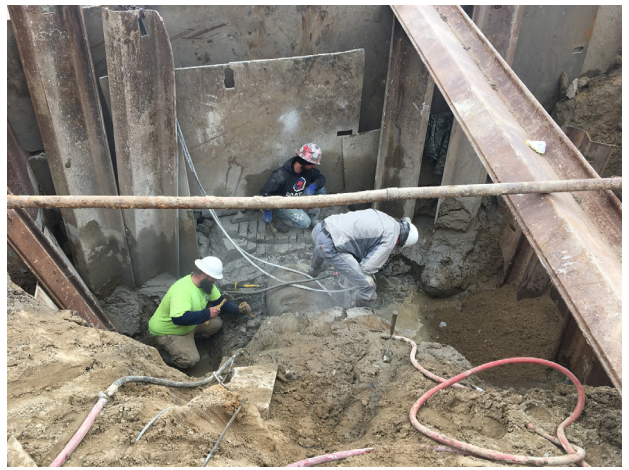
LGC Crew removing concrete encasement from the 24" pipe to install the line stop. Location is Marquette & Inkster, Detroit.
