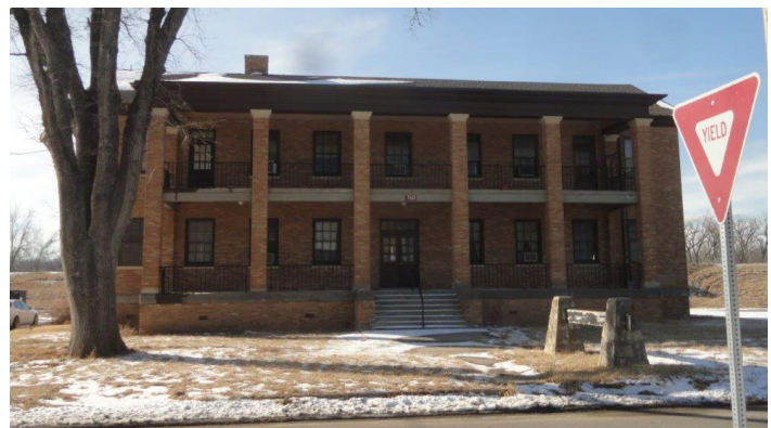
Fort Riley Renovation Project
