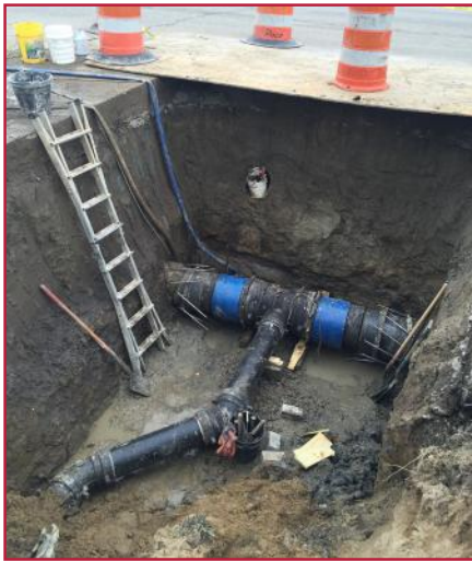
Replacement of Water Main Piping
