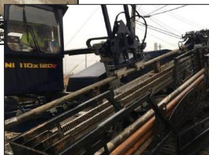
The LGC Global Inc. team studies the site-specific conditions for crossing the staging area, and mobilized work equipment and the directional drilling machine to commence work.
